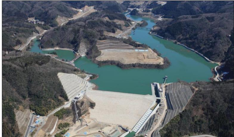
*Figure 1. Aerial photo of Tono Dam and its reservoir. Intake tower can be seen at end of pier to the right of the dam. Photo courtesy of Tono Dam Reservoir Management Office.*
